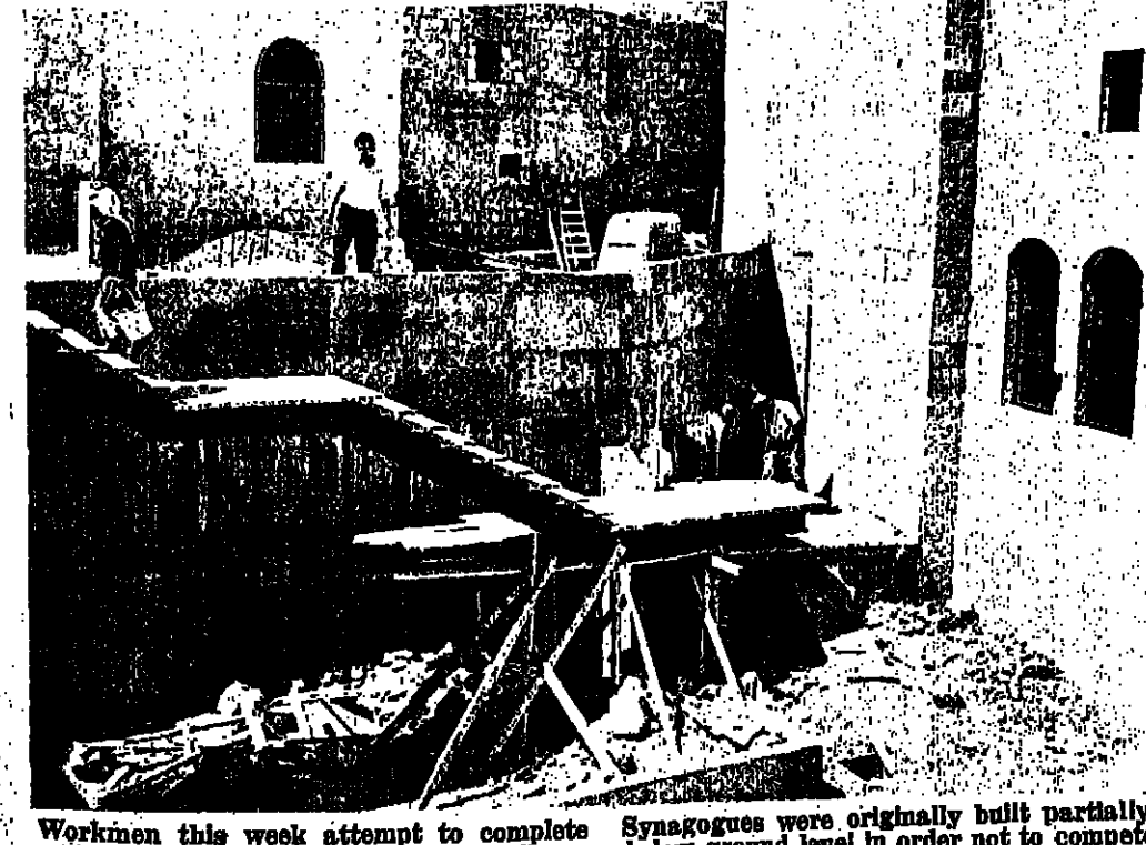
Workers this week attempt to complete main entranceway to the Sephardi Synagogue complex before next week's opening. Synagogues were originally built partially below ground level in order not to compete in height with nearby mosques.
